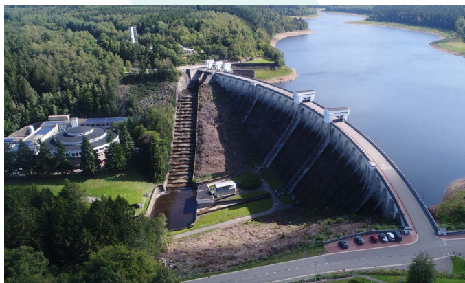
A site under constant control. The spillway, which drains 230 m 3 /s. © PSW MI (DBR)
